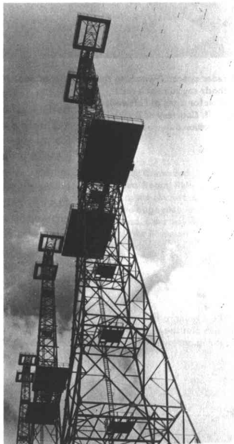
Towers of the RDF system. Their open construction enabled many of them to withstand bomb explosions. Courtesy of British Information Services
